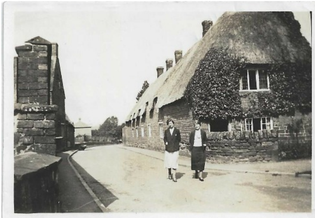
Blue Row, Church Lane - demolished c 1930
